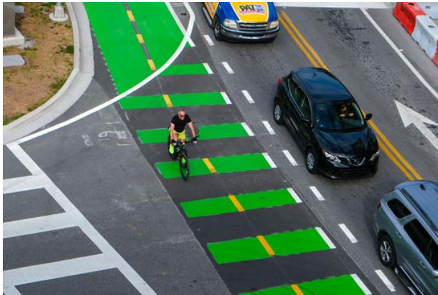
Green cycle track marking along Cass Street: N Boulevard to W of Tyler Street.
